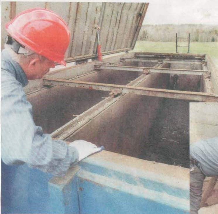
Tri-City dewateres septage in a DeTainer dewatering box supplied by Green Mountain Technologies. At the right, company president Gene Dube takes an effluent sample.
